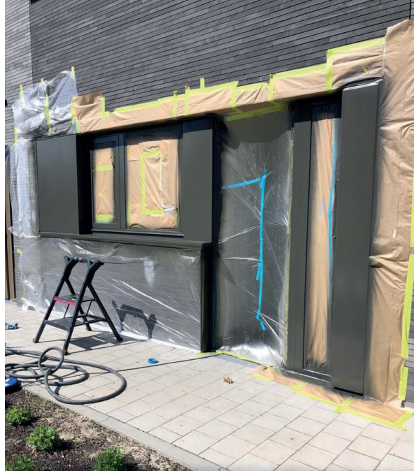
Figure 3.14: Refurbishment by repainting elements on site. © Respirepair
