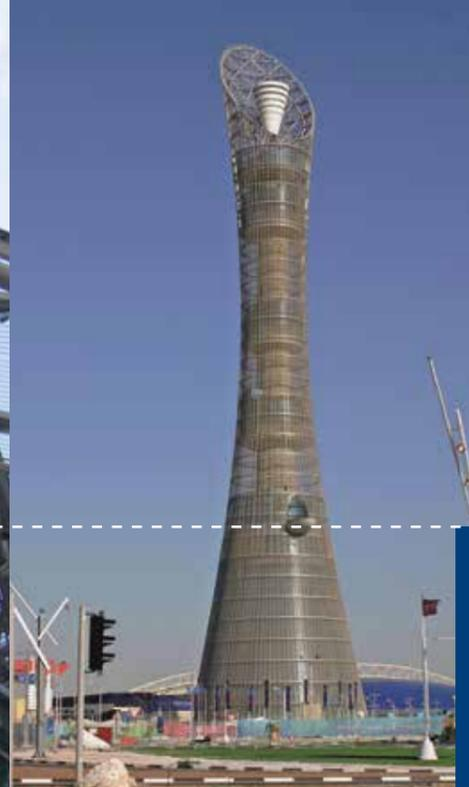
The tower features a double-skin façade, which has been designed to a very high specification by Reynaers Aluminium. To meet the aesthetic and technical demands of the curved architecture, Reynaers Aluminium created bespoke solutions based on its unitised curtain wall system **CW 86** and transom-mullion curtain wall system **CW 50**. Reynaers Aluminium's innovative systems were specified as they are proven to have a great track record, with guaranteed performance even in extreme climates.
